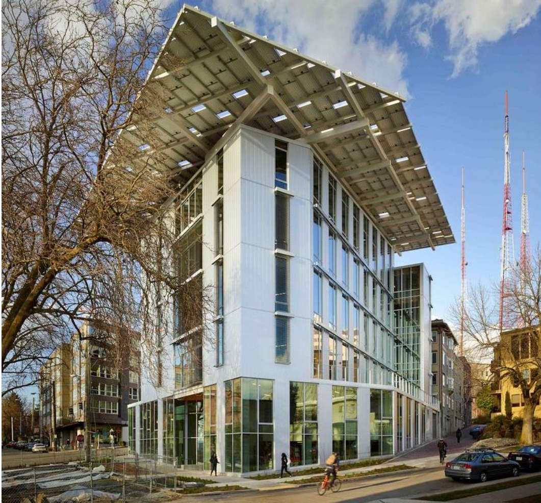
Bullitt Center, Miller Hull, Seattle, USA, 2013
