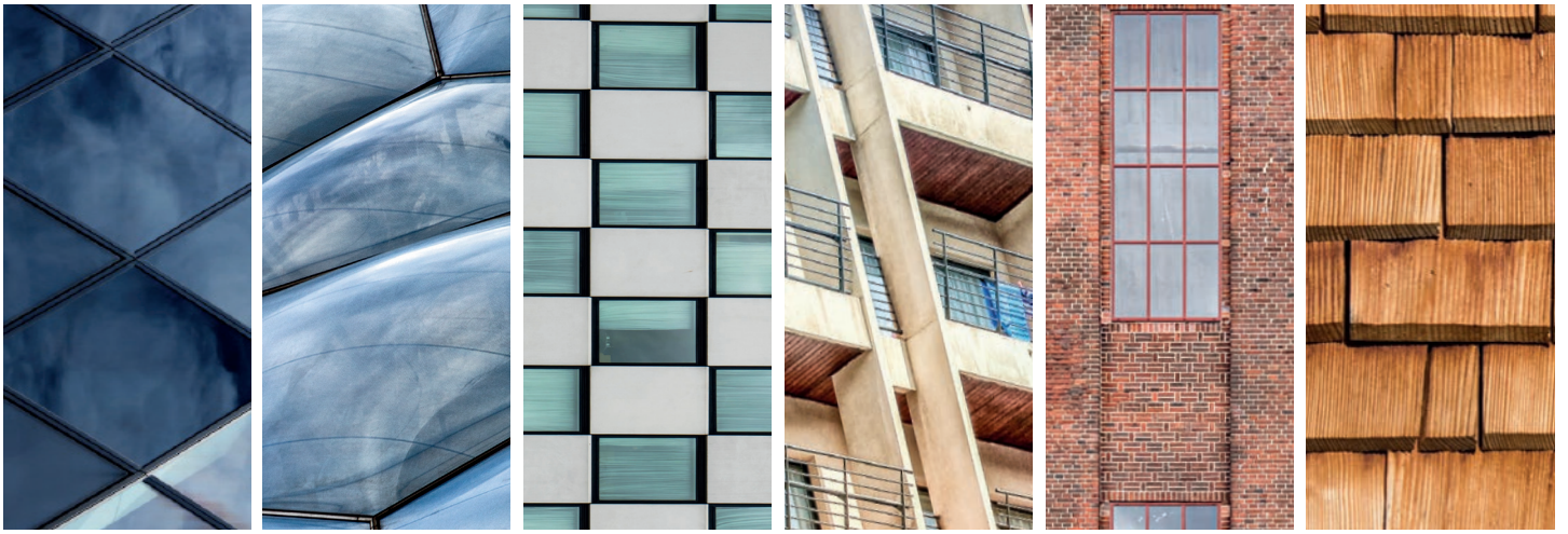
Figure 1.6. Examples of building envelopes. (a) Glass curtain walls, (b) ETFE envelope, (c) Bearing façade made of concrete and glass (c, d), (e) brick facade, (f) wood cladding facade. Credit: Pixabay Licence
